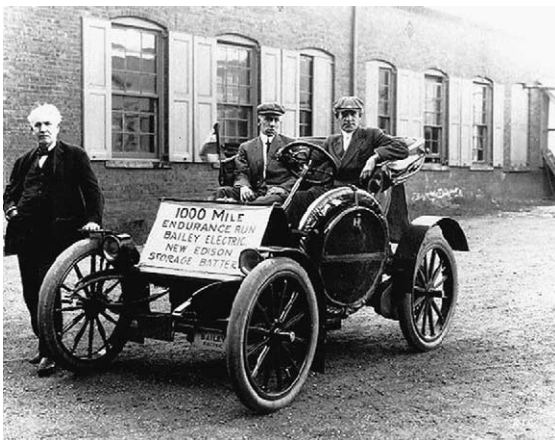
Fig. 18. Endurance test for storage battery.
